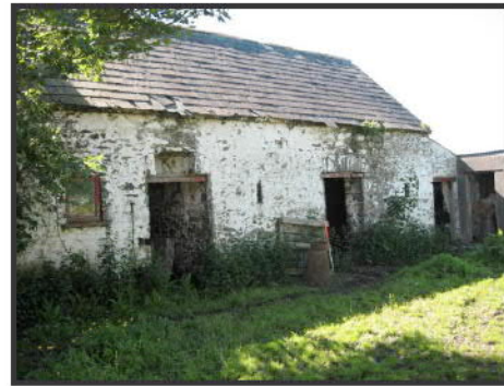
Plate 17: CHS 9; Building 2, east elevation
