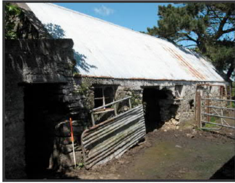
Plate 3: CHS 2; Building 1, southeast elevation looking north
