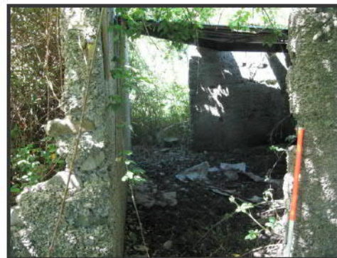
Plate 25: CHS 11; concrete walls of looking W
