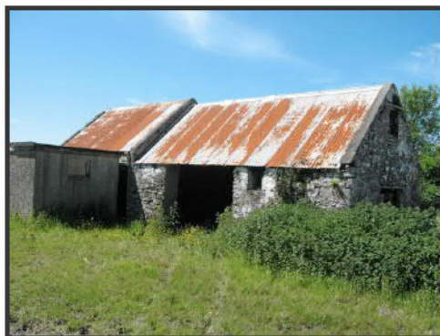
Plate 7: CHS 2; Building 4, southeast elevation, looking northwest
