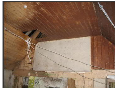
Plate 21: CHS 9, ceiling of Building 4
