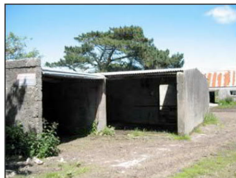
Plate 8: CHS 2; Building 5, north elevation, looking northeast
