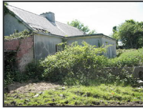
Plate 4: CHS 2; Building 2, northwest elevation, looking south
