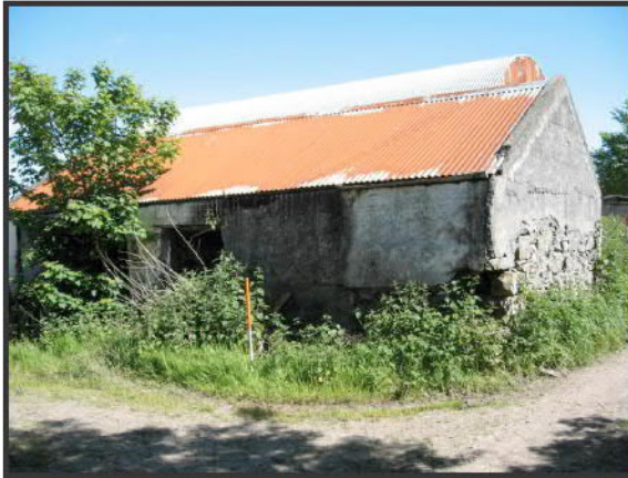
Plate 22: CHS 9; Building 5, from northwest
