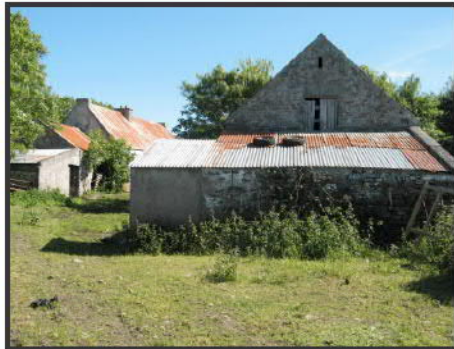
Plate 18: CHS 9; Building 2, north gable
