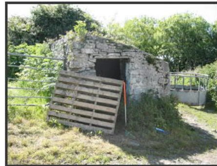
Plate 19: CHS 9; Building 3, east elevation
